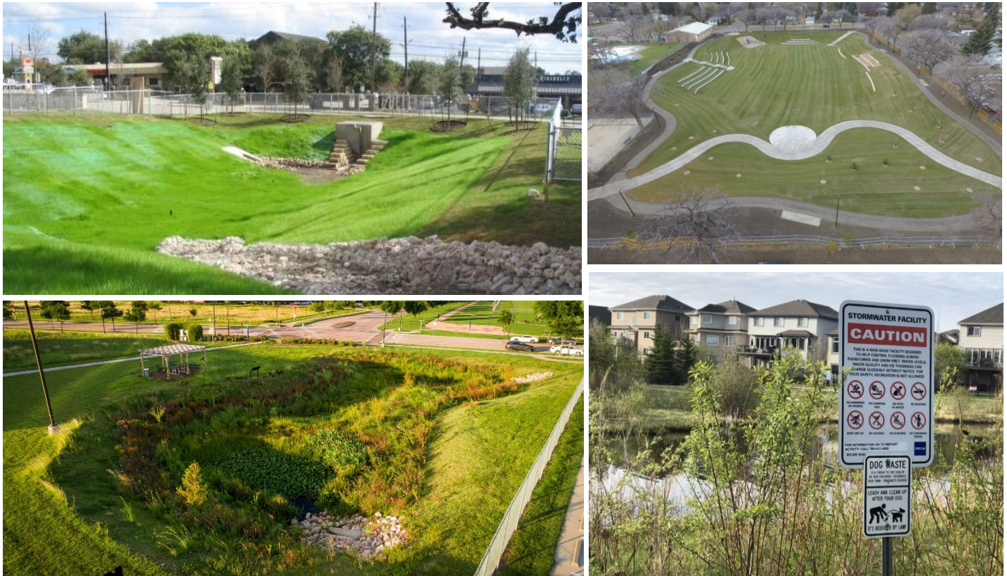
Top Left: Fencing can be installed around a basin’s permitter (City of White House, TN); Top Right: Some basins are designed for dual purposes. This basin is used as a recreational area. (Sacramento State University); Bottom Right: Safety signage installed at a detention basin in Edmonton, AB, Canada (Jolyn Hall, Schmidt Realty Group, Inc. ); Bottom Left: Landscaping can deter people and vehicles from entering a detention basin in Houston, TX (photo: Bryan Malloch).
