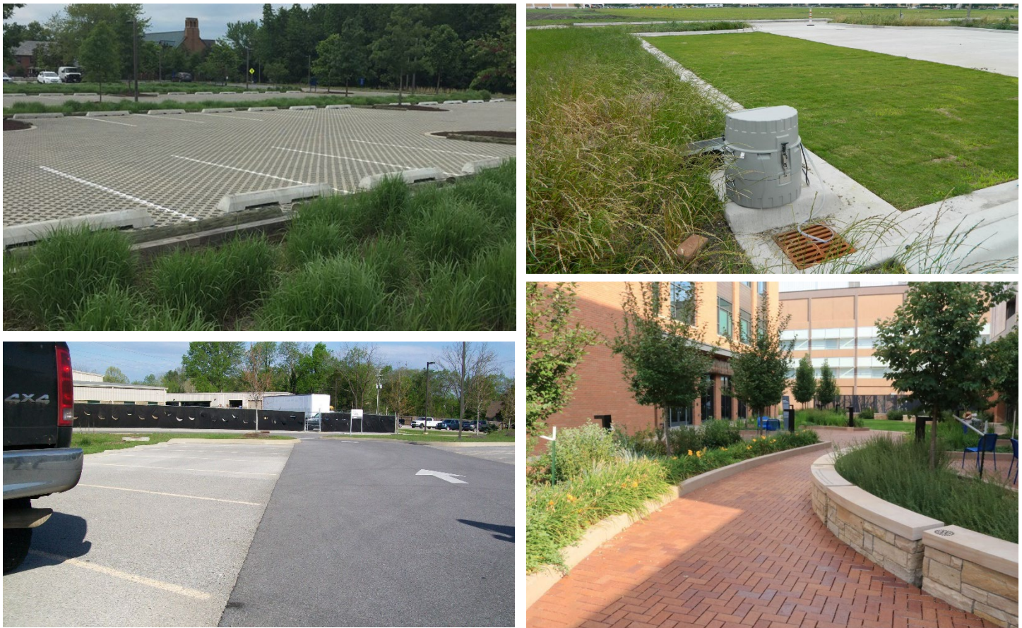
Figure 5.8.2.1 Examples of Permeable Pavement Systems Applications
