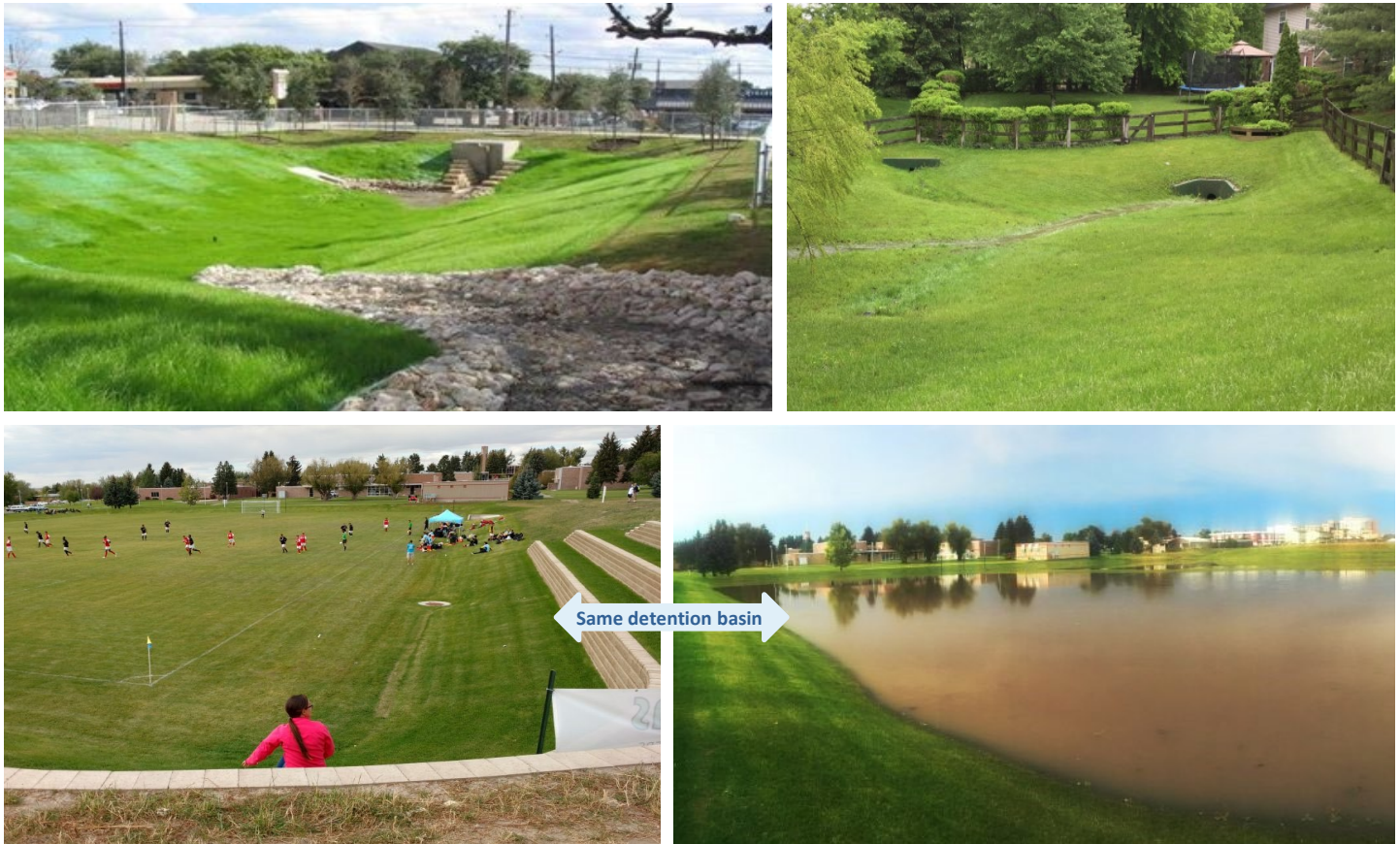
Top left: City of White House, TN; Top right: Clermont OH Soil & Water Conservation District; Bottom left and right: Detention basin used as recreational fields in Great Falls, MT during a dry period (left) and after a large storm (right), TDH Engineering.
