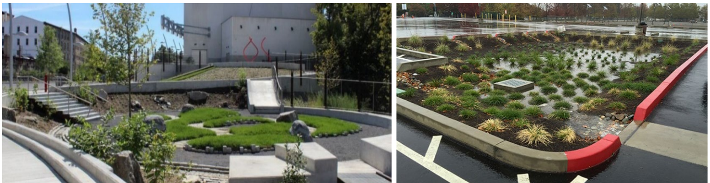
Left: Pathways along and through a bioretention area guide pedestrians to appropriate places to walk (City of Philadelphia, PA Water Department); Right: Concrete curbing around a parking lot bioretention area keeps vehicles and people out while allowing stormwater in (Sacramento State University);
