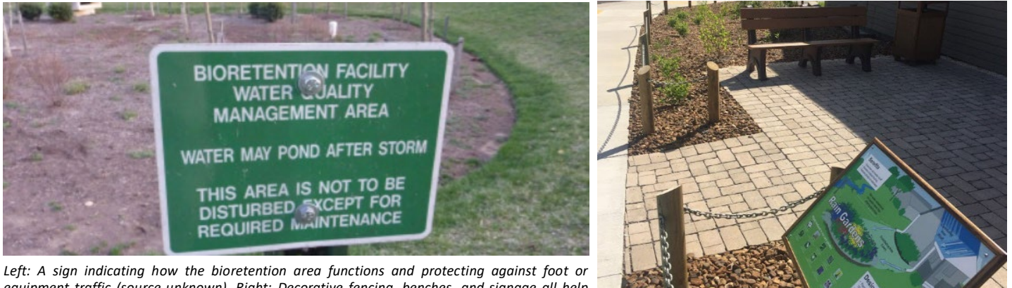
Figure 5.1.8.2 More Examples of Bioretention Area Protection
