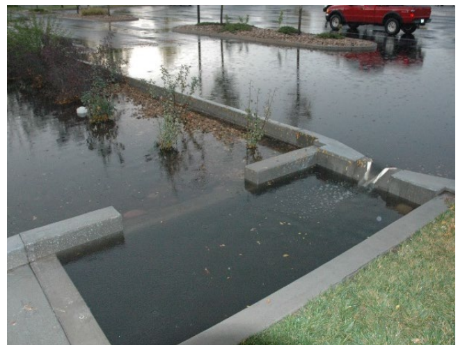
Figure 5.16.5.1 Example of a Pretreatment Forebay (Source: Urban Water Center)
