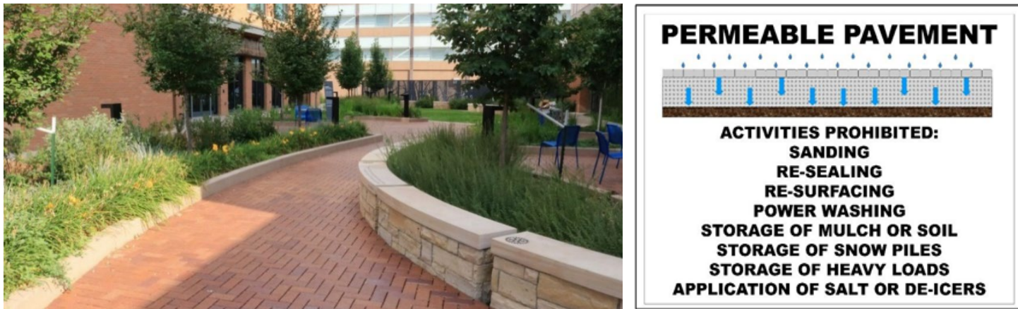
Left: Permeable pavement can be landscaped so that barriers, like curbing and walls, keep mulch, sediment, and plant debris within pervious areas. (Source: City of Boulder CO); Right: Example layout for a sign to be located at a permeable pavement (Source: NCDEQ Stormwater Design Manual)
