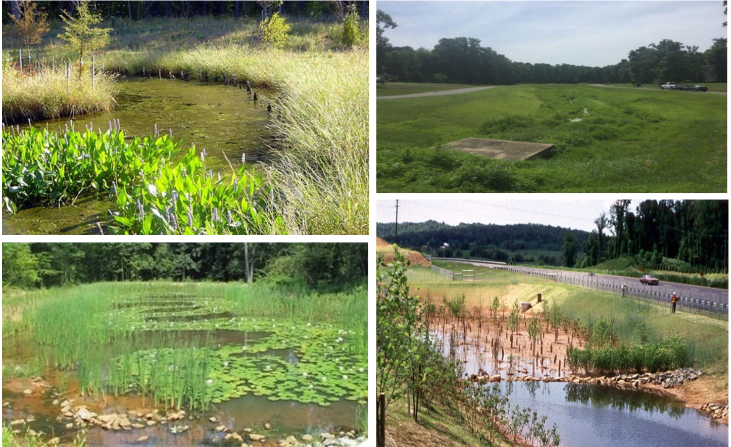
Top left: Shallow wetland (Maryland Department of Transportation); Top right: Extended detention shallow wetland (Maryland Department of Environment); Bottom right: Basin/wetland system (Connecticut Stormwater Quality Manual); Bottom left: Pocket wetland (Athens-Clarke County, GA)
