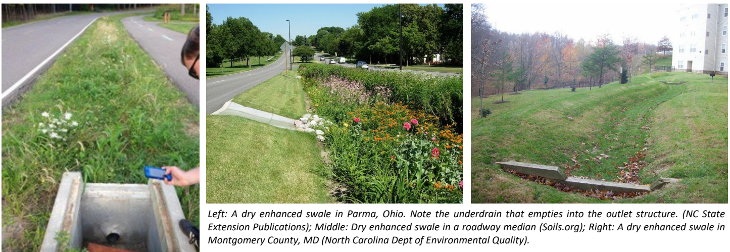
Figure 5.3.2.1 Examples of Dry Enhanced Swale Applications
