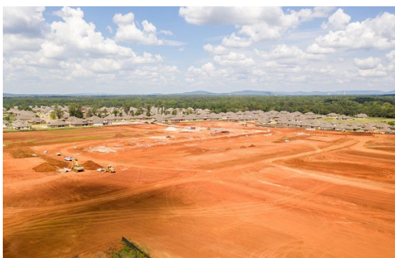
Figure 4.5.6.1 Examples of Mass Grading and Site Footprinting
