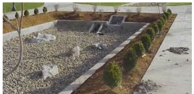
Left: Schematic of a surface sand's filter basic components (Source: GDOT Drainage Manual, 2023); Right: Sand filter bed of a surface sand filter (Source: NCDEQ Stormwater BMP Manual).
