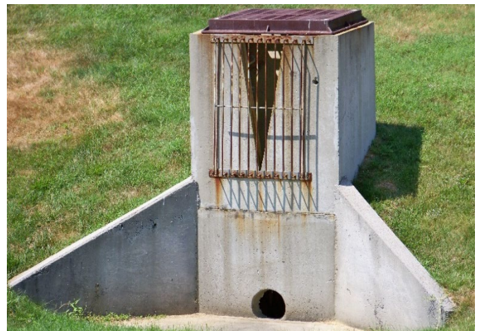
Figure 5.4.1.2 Example of a Multi-Stage Outlet Structure
