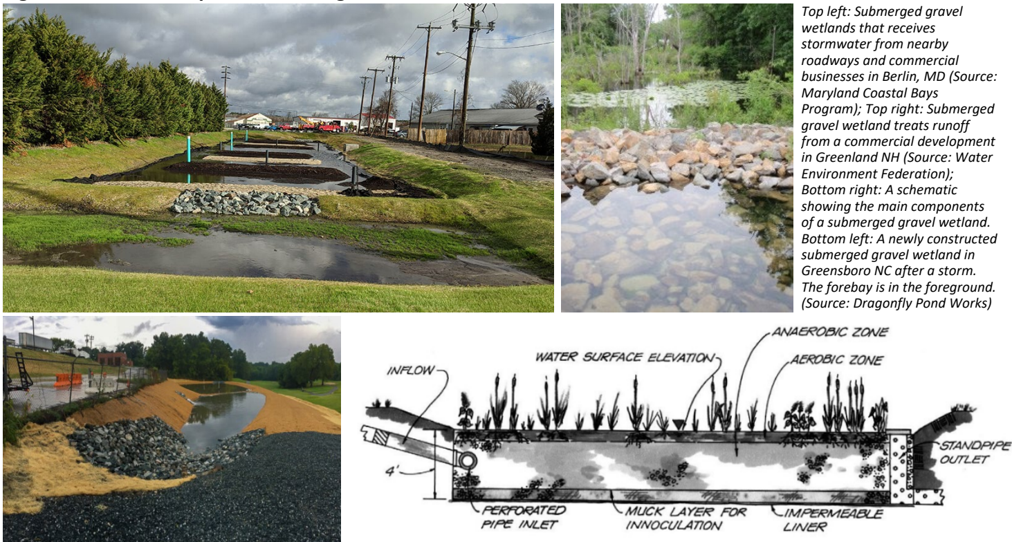
Figure 5.11.2.1 Examples of Submerged Gravel Wetlands
