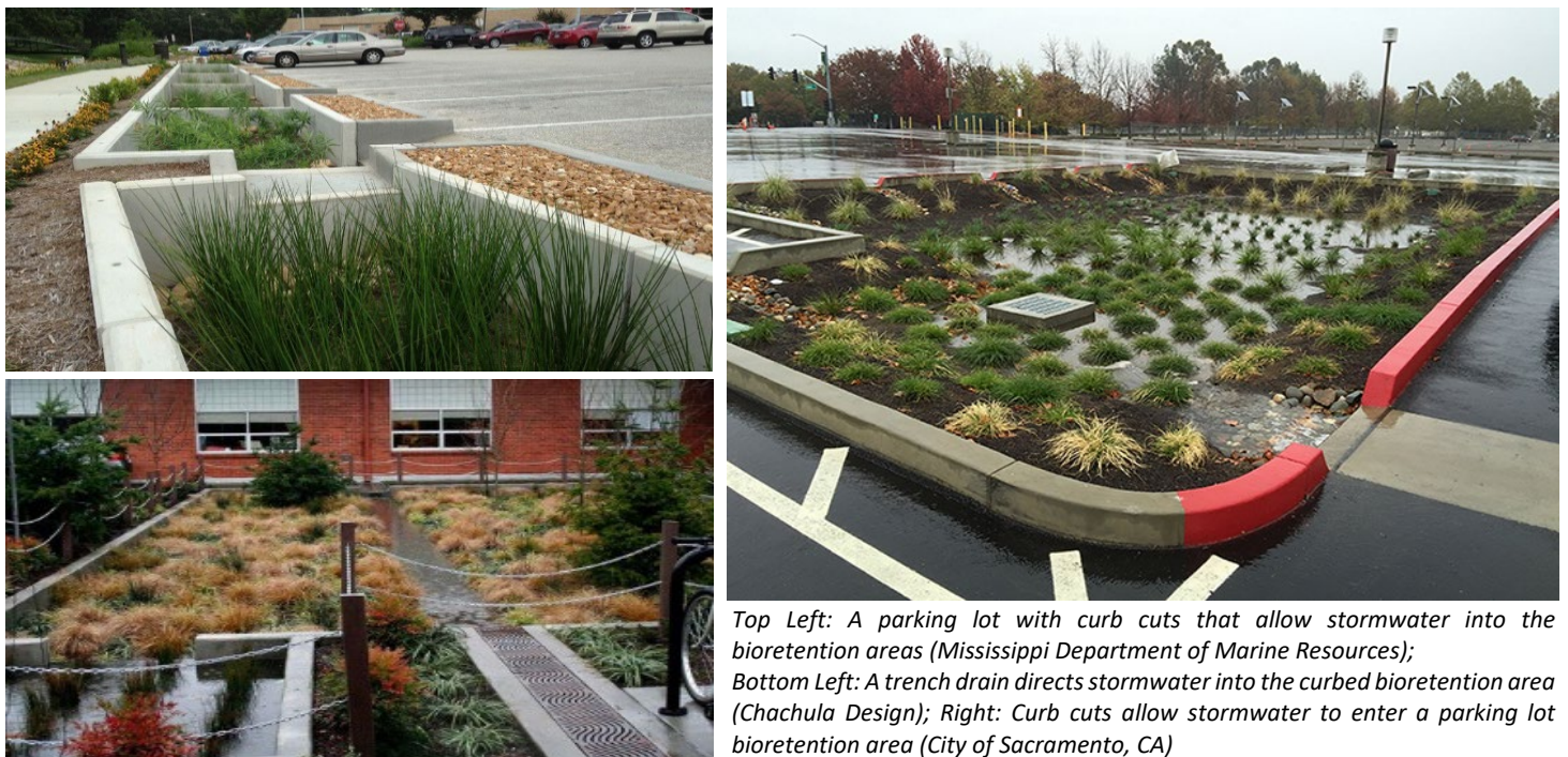
Figure 5.16.2.2 Examples of Different Curb Cut Designs
