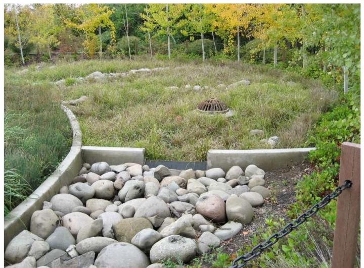
Figure 5.16.8.1 Rock Forebay (Source: Water Conservation Technologies)
