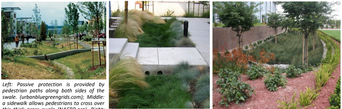
Figure 5.3.8.1 Examples of Dry Enhanced Swale Protection Measures
