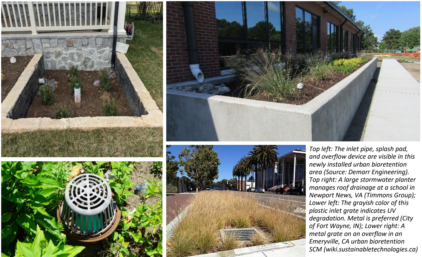
Figure 5.13.5.2 Examples of Inflow and Overflow Structures
