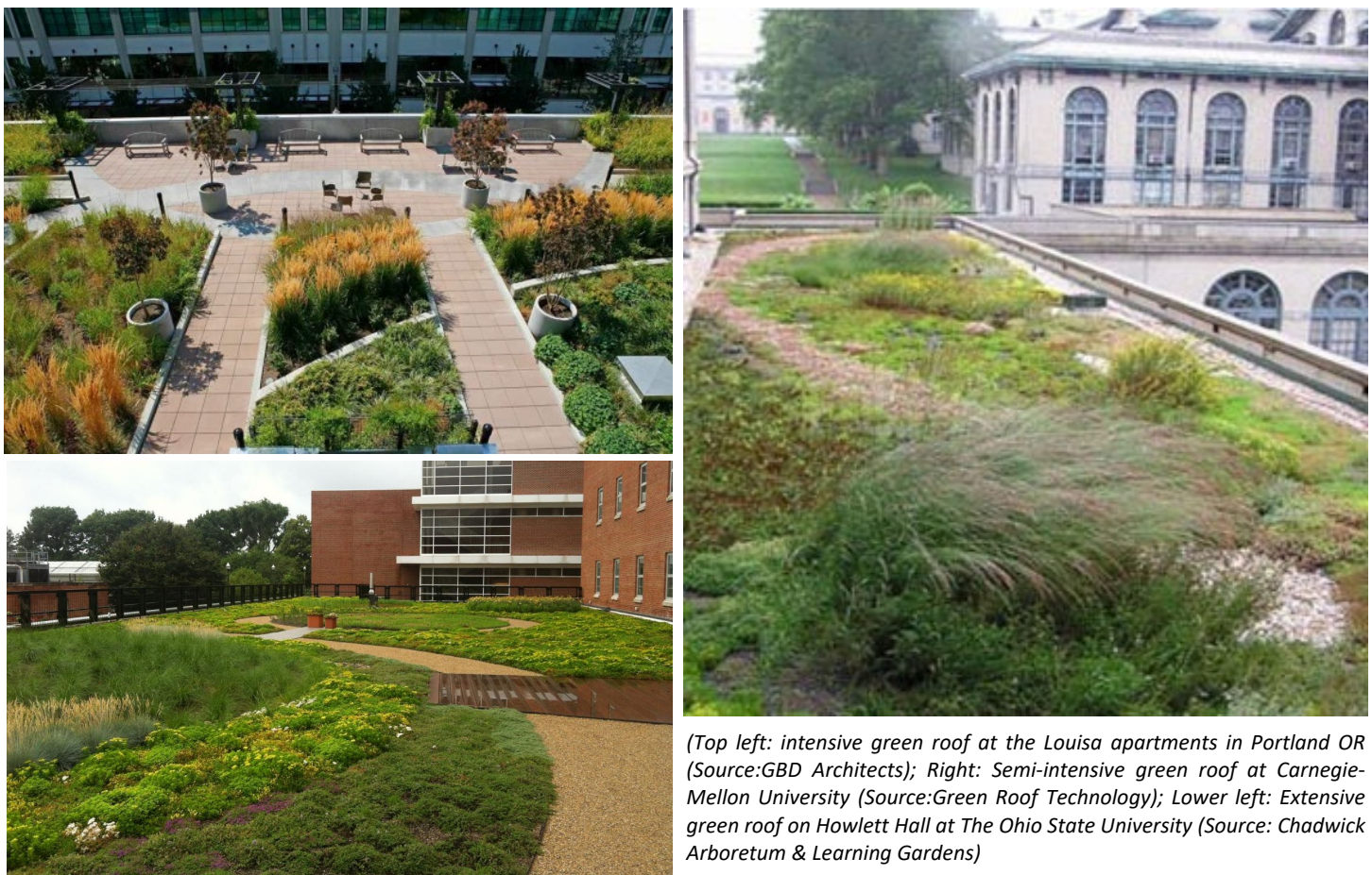
Figure 5.5.2.2 Examples of Intensive and Extensive Green Roofs
