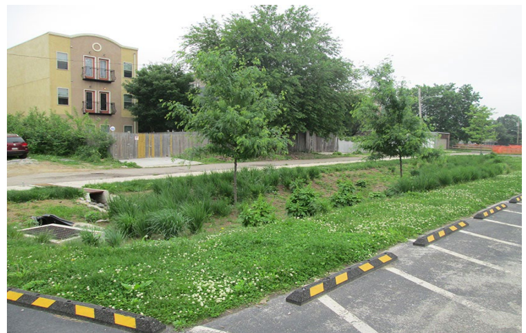
Figure 5.16.9.1 Example of Grass Filter Strip
