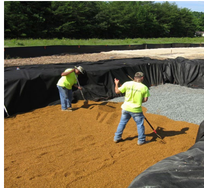
Figure 5.1.10.1 Examples of Good Installation Practices for Bioretention
