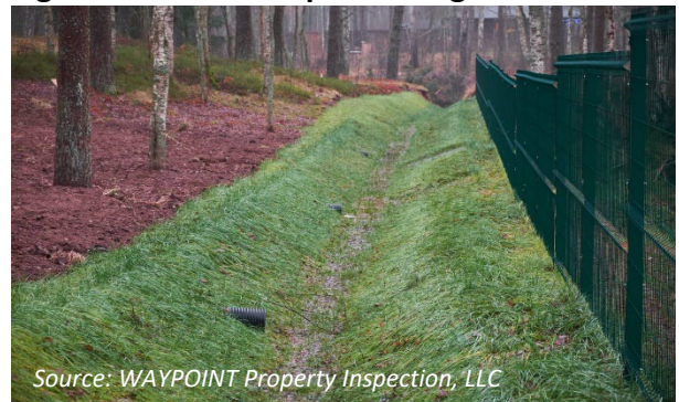
Figure 4.7.2.1 Examples of Vegetated Swales
