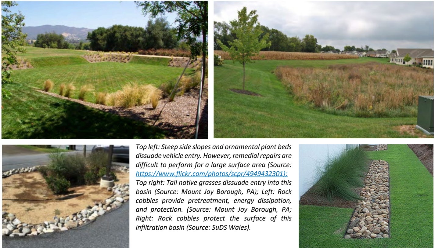
Figure 5.6.8.1 Examples of Infiltration Basin Protection
