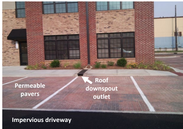
Figure 5.8.2.1 Permeable Pavement Systems and Run-on
