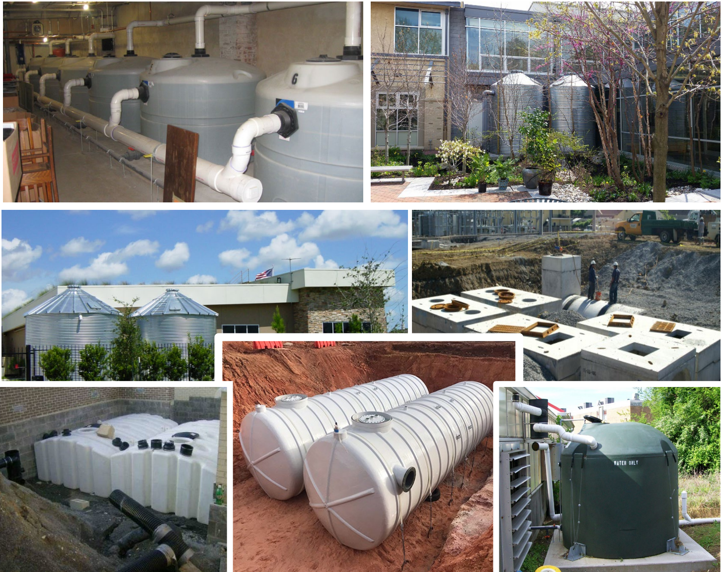
Top left: Surface cisterns in Philadelphia, PA, Philadelphia Water Department; Top right: Subsurface cistern system in Philadelphia, PA, Philadelphia Water Department; Middle left: Galvanized steel (Source: Protank ); Middle right: Multiple precast concrete units (Source: unknown); Bottom left: Polyethylene Modular Units (Source: VADCR, 2011); Bottom middle: Fiberglass units (Source: Rain Harvest Systems ); Bottom right: Polyethylene tank (Source: Knox County, TN)
